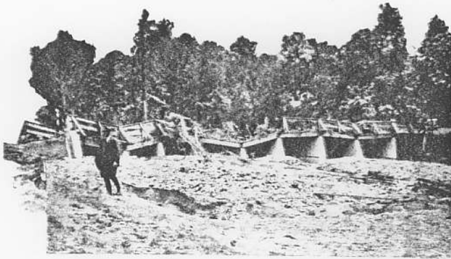
In these two snap-shots may be found evidence of the necessity for comprehensive engineering survey of the water shed through which a good road may be built. In one of these structures in Garland county an effort was made by the local authorities to economize both in engineering and in material, with the result that the first heavy rain, coming two months after completion, totally demolished the structure. A proper engineering design, recommended by the Insiders for a better construction, would have saved the total investment.
