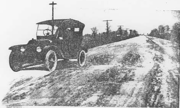
A section of the Arkansas-Louisiana Highway, north of Grady in Lincoln county, showing deterioration resulting from a faulty sub-grade on gumbo soil. This section is being re-constructed under the provisions of the Harrelson Act, a base of hard clay and sand being substituted for the gumbo and attention given to proper drainage with the constant maintenance patrol of the road, under the future operation of the Harrelson Act. No further deterioration will be allowed to reach such a stage as that shown in the picture.
