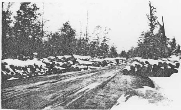
A section of the Arkansas-Louisiana Highway, north of Grady in Lincoln county, showing deterioration resulting from a faulty sub-grade on gumbo soil. This section is being re-constructed under the provisions of the Harrelson Act, a base of hard clay and sand being substituted for the gumbo and attention given to proper drainage with the constant maintenance patrol of the road, under the future operation of the Harrelson Act. No further deterioration will be allowed to reach such a stage as that shown in the picture.
